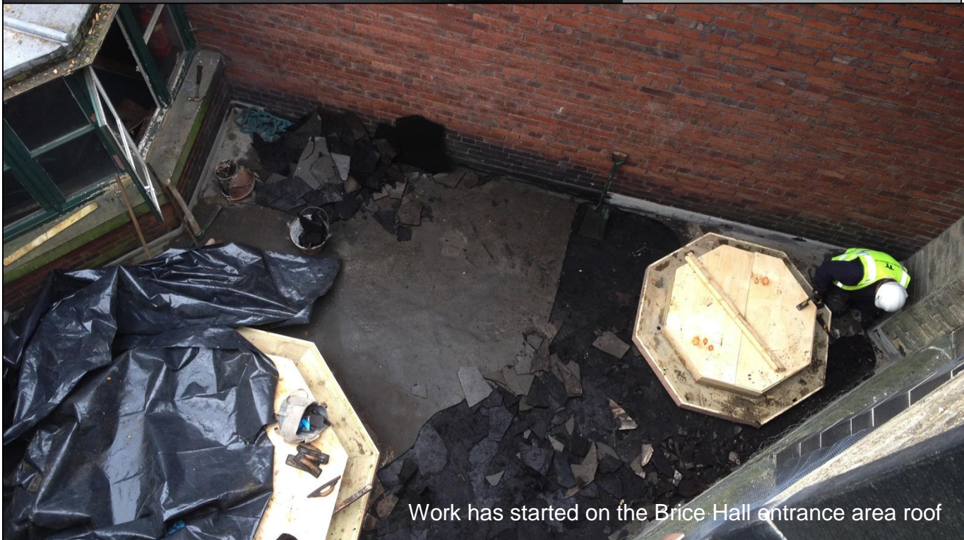
A lovely new roof with painted buttresses and upstands!
