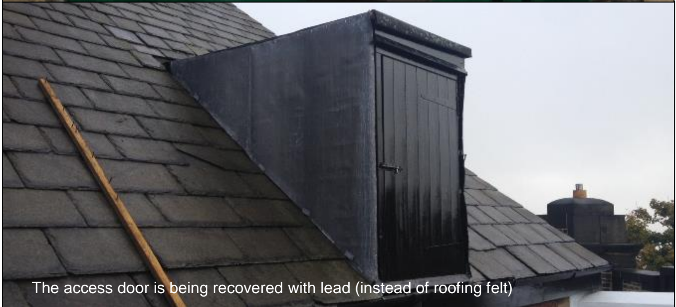
The cupola is nearly completed, with more lead covering being installed
